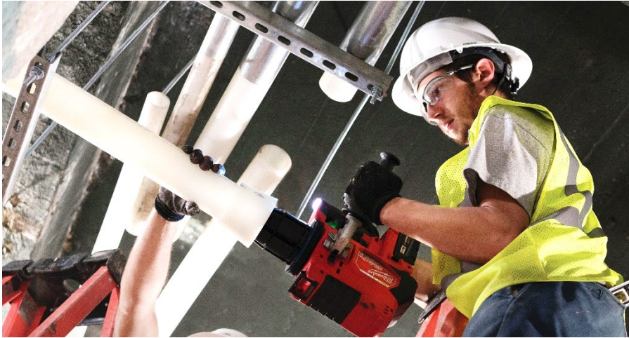
Cold-expansion PEX fittings (brass or polymer) per ASTM F1960
