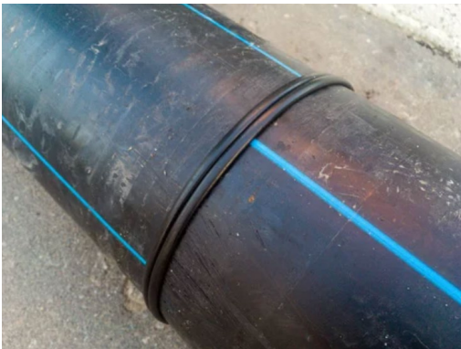
Butt fusion joint
